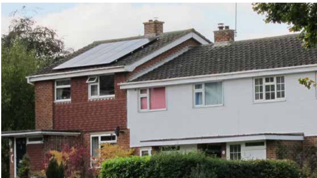
Local House with solar panels
